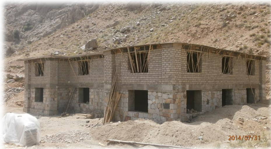
Figure 5: Front view of the school dated 31-07-2014.
