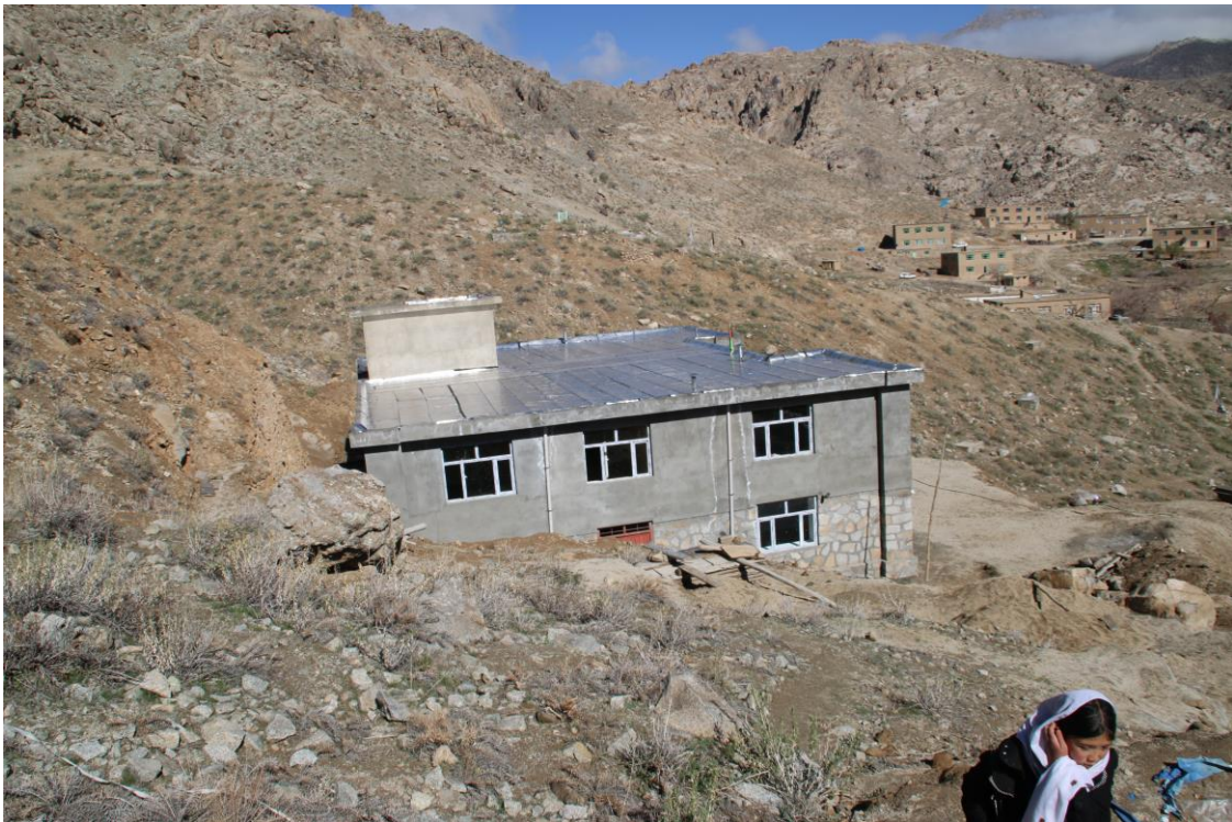
Figure 5: View of the roof of the school
