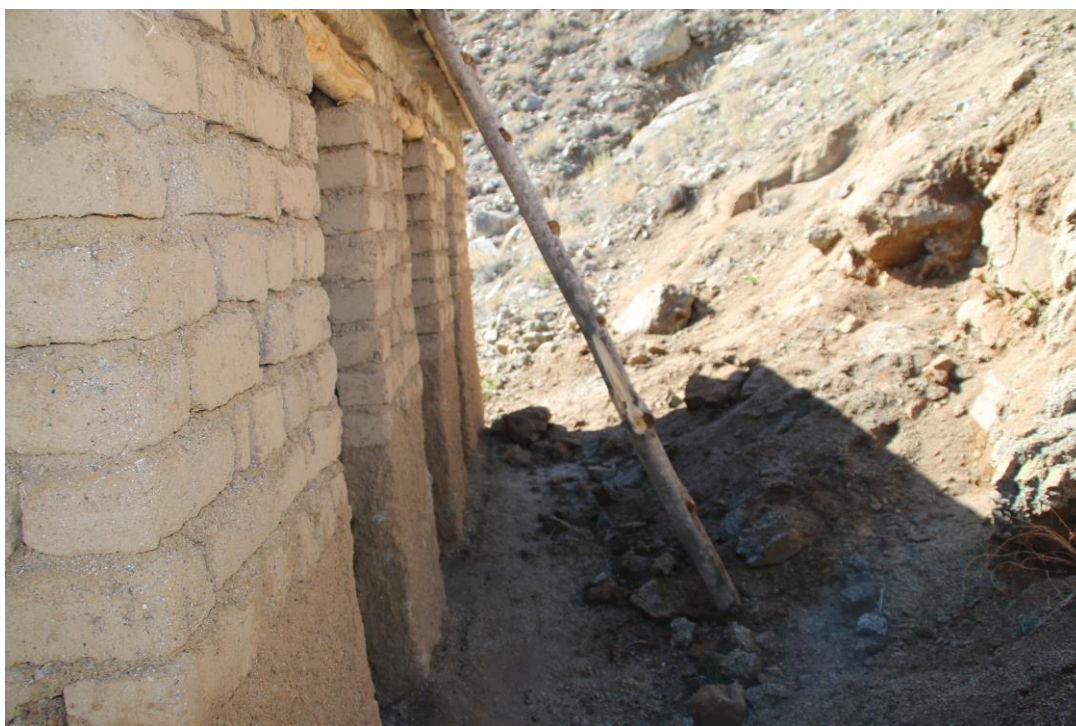
Figure 4: Front of the three toilets
