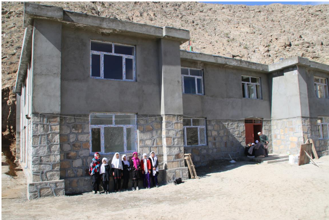
Figure 7: Front view of the school
